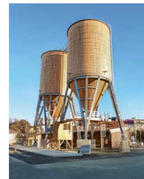
Two log silos in Vienna, each with a capacity of 500 m 3 .
