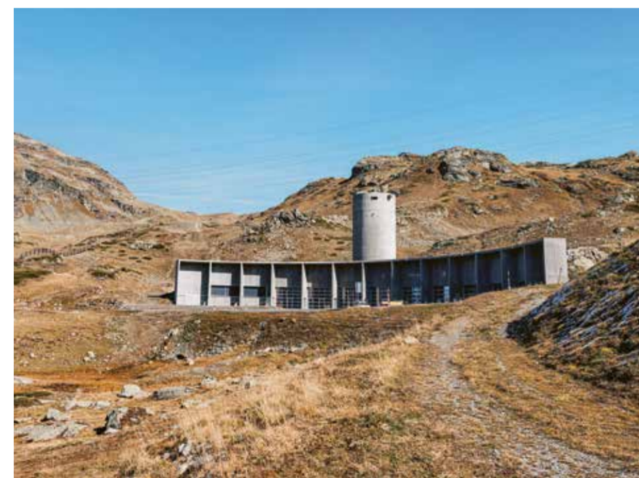
Above: Thanks to its semicircular construction, the maintenance support point blends optimally into the natural terrain.
