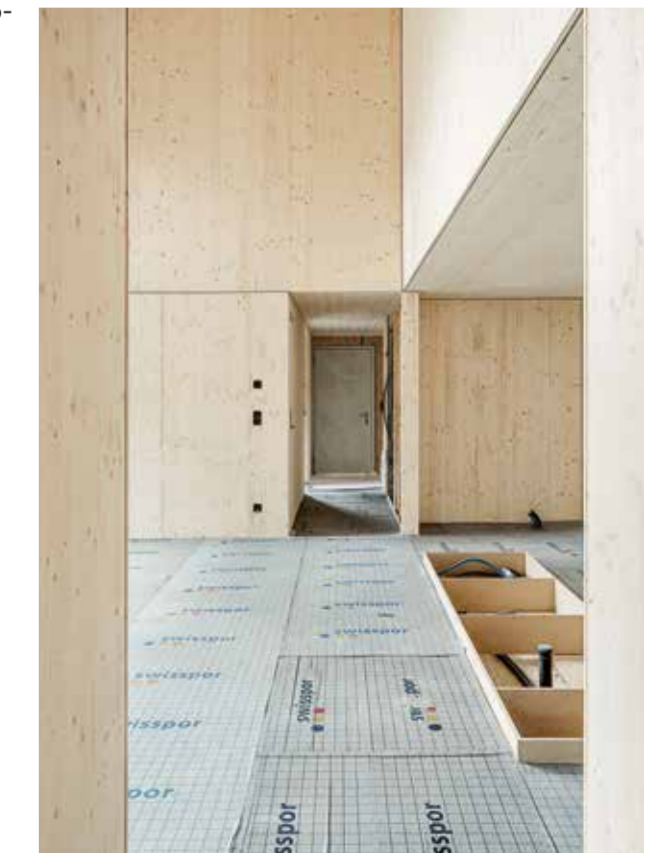
Three-ply spruce cladding dominates the interior finishing.
