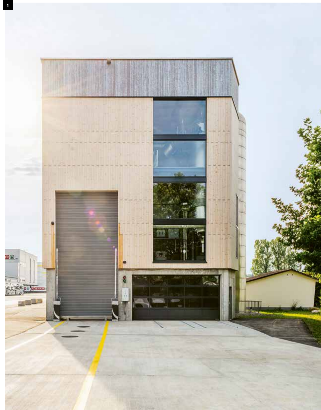
1 The new-build energy plant in Gossau featured a vertical spruce facade treated with UWood®. After around 11 months of weathering with wind, rain and sun, the verdict is extremely positive. 2 Left: untreated facade in rough-cut spruce wood, 11 months after assembly. Right: facade treated with UWood® during the same period. 3 Facade treated with UWood® compared with a pre-aged facade in spruce, which somewhat resembles the natural greying.
