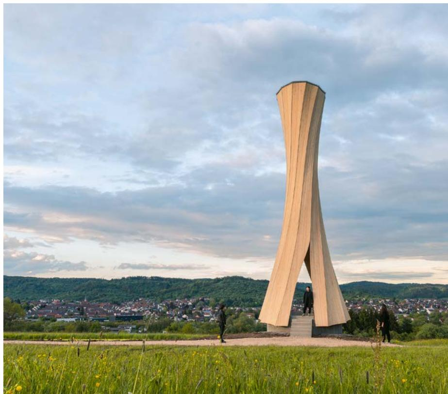
Until now the manufacture of curved wood has been an energy-intensive, mechanical reshaping process requiring heavy machines. A new research study by Empa/ETH Zurich and the University of Stuttgart represents a paradigm change: flat timber components curve themselves into a pre-defined shape without mechanical means in a controlled drying process. Crucial in this process are the amount of moisture removed and the make-up of the layers in the component.
