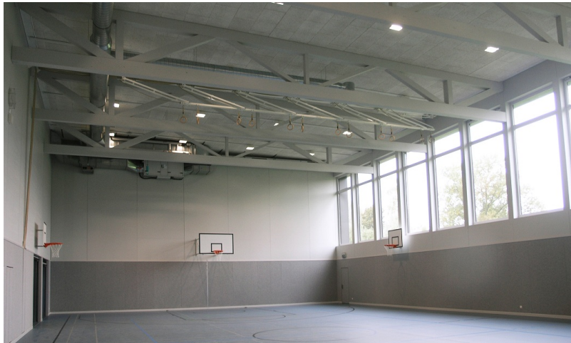
Temporary prefabricated construction
