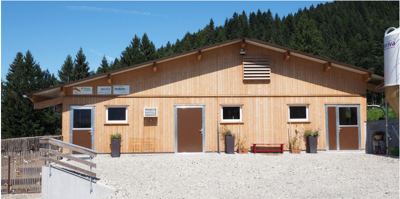
Front side with spruce/pine cladding
