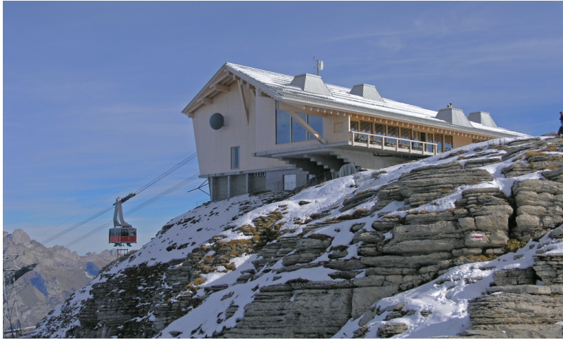
South-west view of the mountain restaurant
