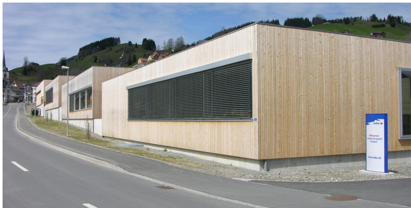
Building complex next to the road
