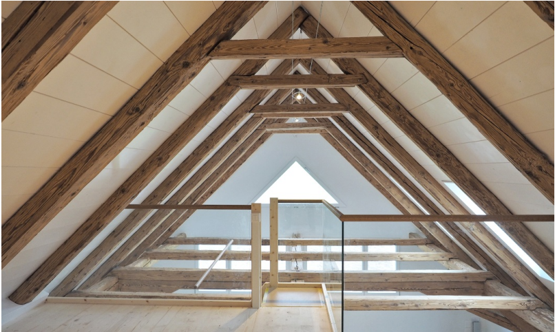
Roof truss, renovated and remodelled
