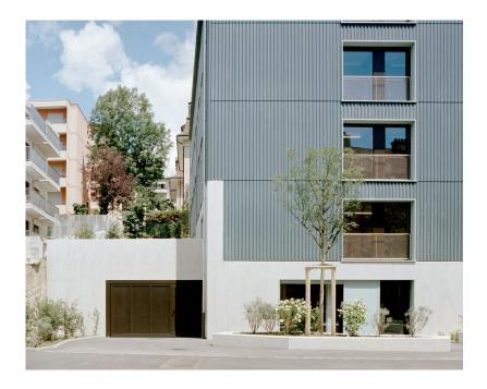
The building was designed as a timber structure with a facade and roof made of corrugated eternit.
