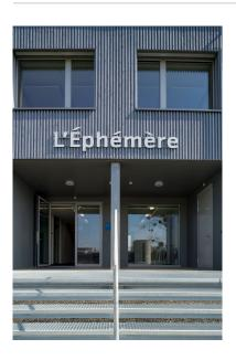
The name of the temporary office building is L'Éphémère, meaning transience. Yet the temporary structure with its vertical timber facade made of spruce and fir does not look makeshift, but instead of very high quality.
